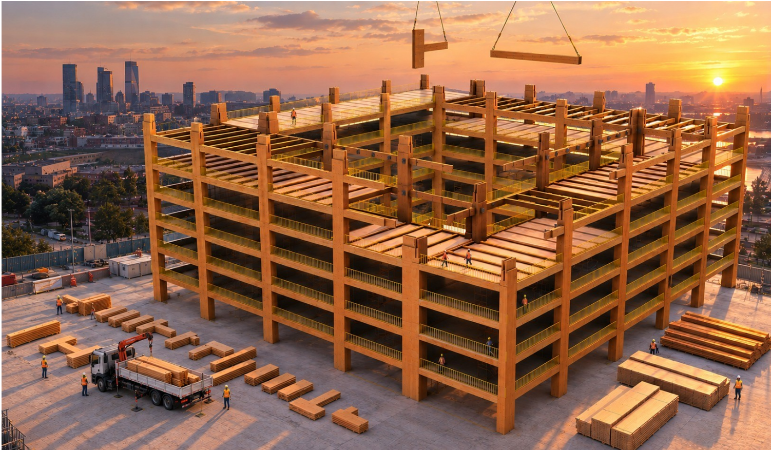
Concept render: flagship project site, modules and purlins placed dry, guardrails only and no scaffolding.
